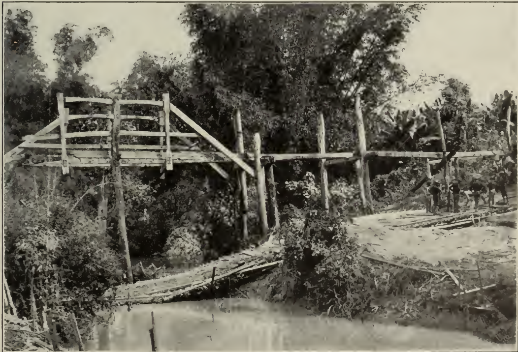
BRIDGE STRIPPED OF FLOORING BY RETREATING INSURGENTS; FORD PREPARED BY ENGINEERS.
